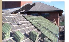
During the reinstallation, new battens and additional insulation were installed.
