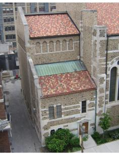
The custom copper gutters were replaced and the tiles reset.
