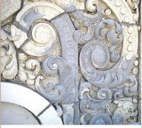
Here the damage to the highly ornamental main cartouche has been carefully repaired and is ready for reglazing. Custom repair materials were by Edison Coatings.
