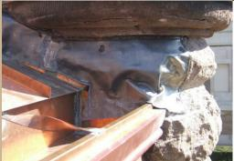
The design of the building required creative material use and design, as with this lead sheet flashing against the irregular curved granite at the end of the gutter.
