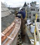
Over 400 feet of custom, double-walled copper gutter – including this extensive curved section – was fabricated from sheet stock in our shop, and installed.
